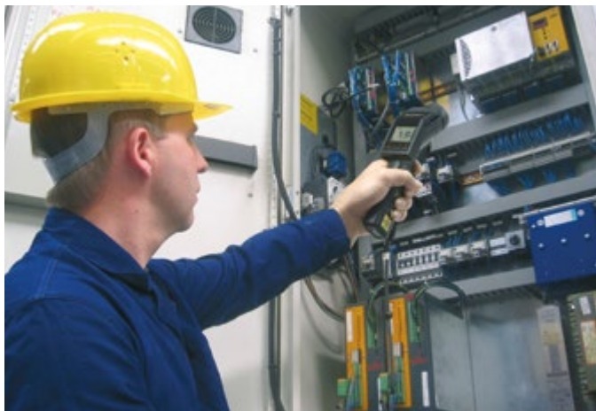
Detailed infrared temperature measurement of an electric control with the help of the installed close focus optics for 1 mm ranges of the optris® LS
